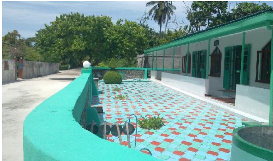
Sh.Narudhoo: Paving of Mosque courtyard
