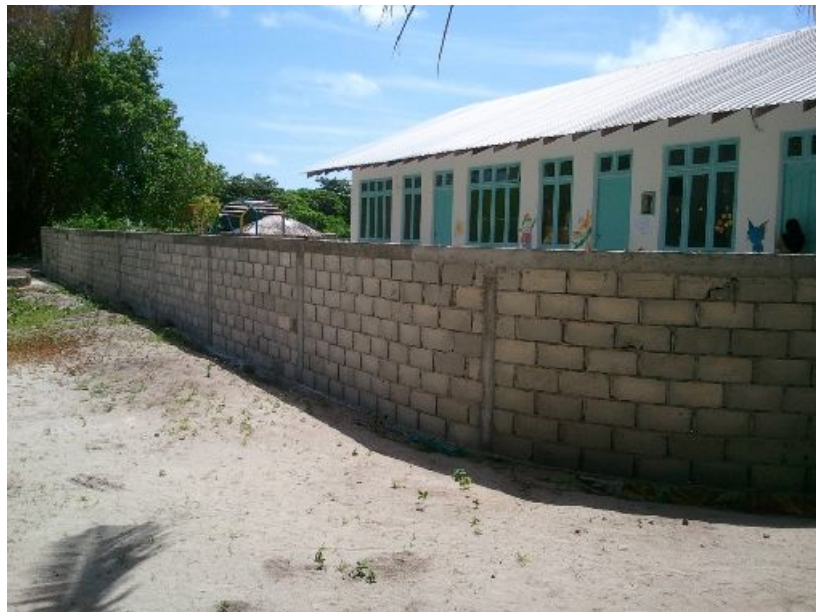
Sh.Goidhoo: Construction of boundary wall for pre-school
