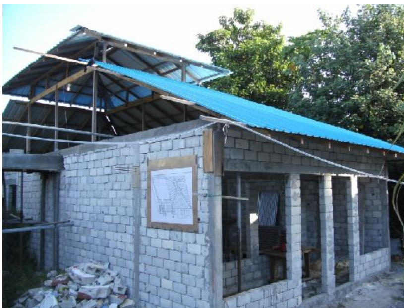
N.Henbadhoo: Construction and roofing of roofing multi-purpose building
